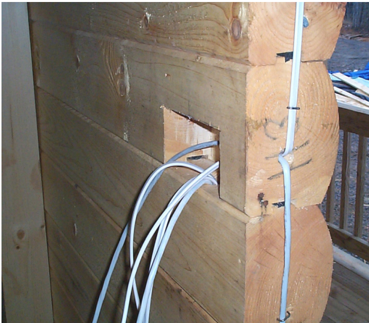
The builder will drill large holes that line up vertically through several rows of logs in order to pull the wiring up through.
