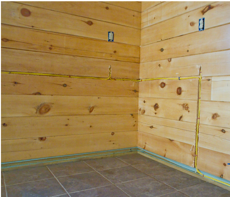
These two examples illustrate an alternative method of installing wiring behind kitchen cupboards. Because of the permanent damage to the wood in this method we suggest you have complete confidence in the placement of the cupboards both now and in the future.
