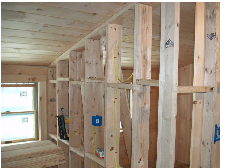
It's an easy thing to hide wiring for switches and outlets in the interior partition walls. Note the drilled holes and secured wiring along the studs.
