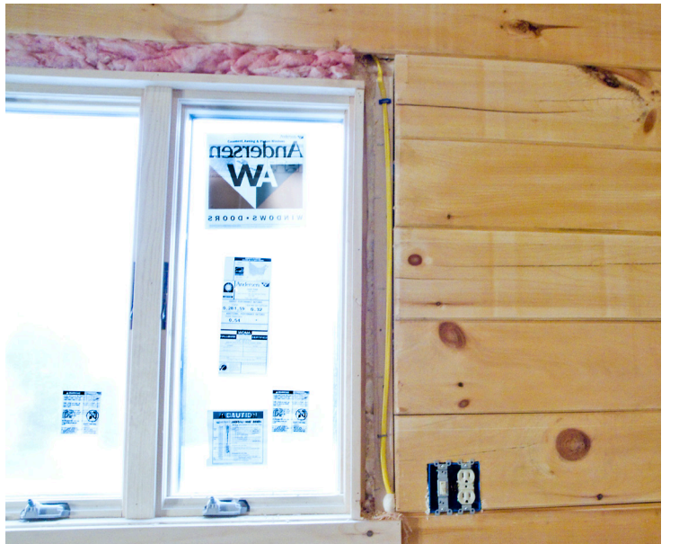
In this example the builder took advantage of the window opening in order to carry the wiring into other regions of the home.
