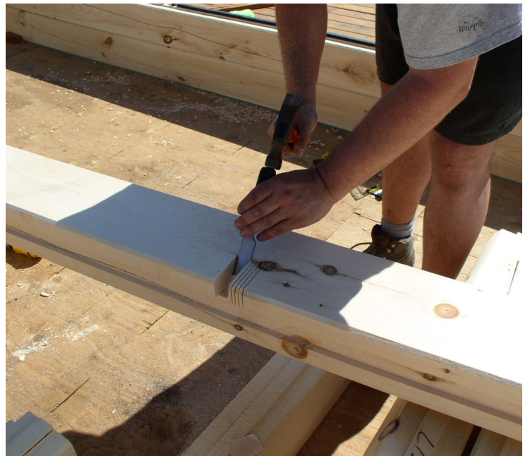
Several closely spaced saw cuts are made to allow a chisel to create a notch to accommodate an electrical outlet.
