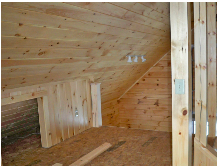
Drilling and notching methods mentioned previously were implemented for the light switch installed on this 6x6 post.
