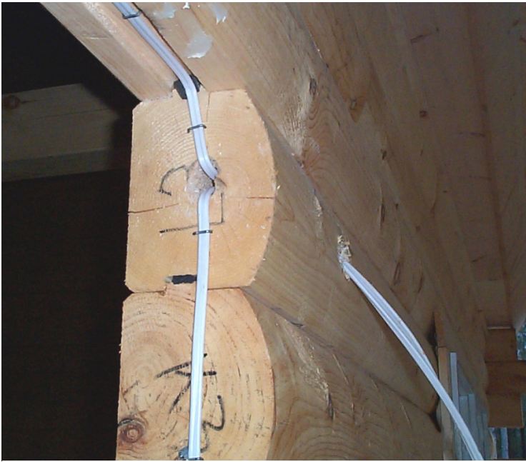
A wall-mounted fixture is prepared by drilling a large horizontal hole and a perpendicular hole to meet it in order to thread the wiring through.
