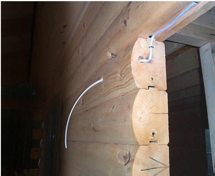
Secure the cable along the center of the door opening and avoid puncturing the wiring with nails when installing the door casing.
