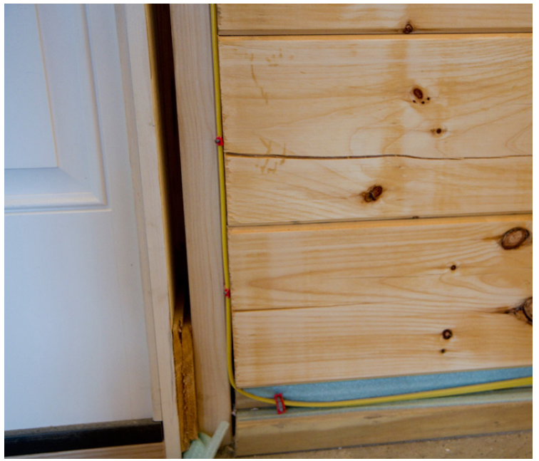
When building on a slab the log rows are started on a 2x4 sitting atop a sill board. The groove created hides the wiring very nicely.
