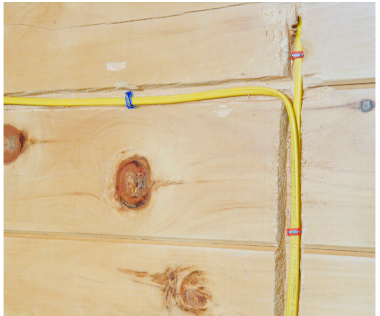
These two examples illustrate an alternative method of installing wiring behind kitchen cupboards. Because of the permanent damage to the wood in this method we suggest you have complete confidence in the placement of the cupboards both now and in the future.
