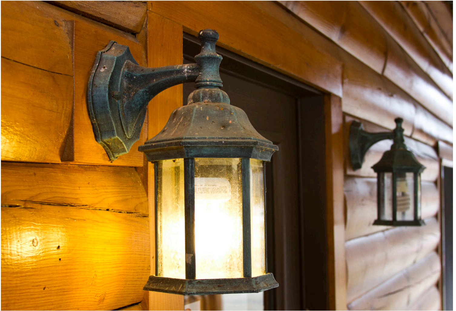
Note the attractive look of this set-in mounting board. It is vertically level and flush with the curve of the exterior wall as is the door casing.
